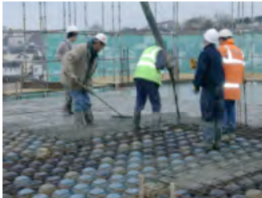
Pouring, Vibrating & Floating Site Concrete
