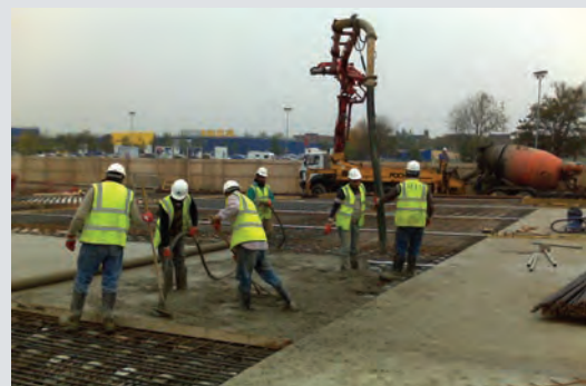
Pouring, Vibrating & Floating Site Concrete
