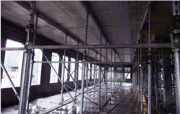
Typical arrangement of props and propping beams
