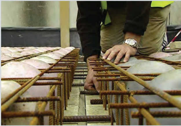
Sliding bottom splice bar central over joints
