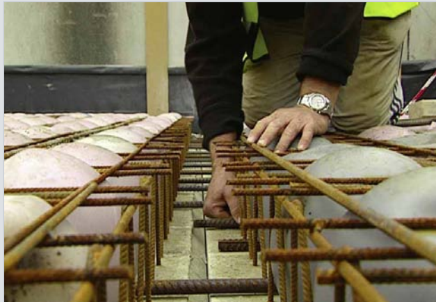
Sliding bottom splice bar central over joints
