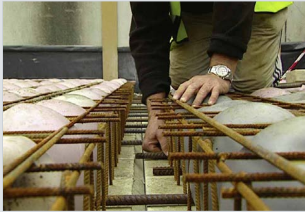
Sliding bottom splice bar central over joints
