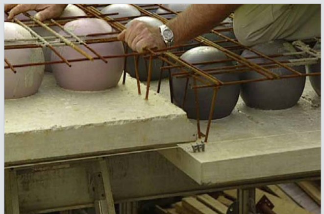
Aligning bubbles between elements
