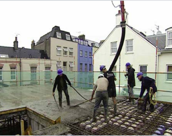
Pouring, Vibrating & Floating Site Concrete
